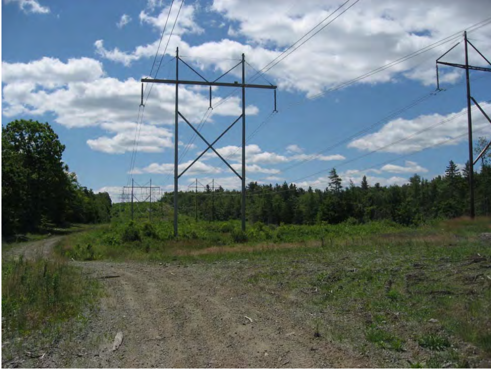
View of existing access road that was utilized by crew in the vicinity of Structure 220. Crews avoided a mapped polygon of Northeastern Bulrush ( Scirpus ancistrochaetus ), a state and federally listed endangered species.
