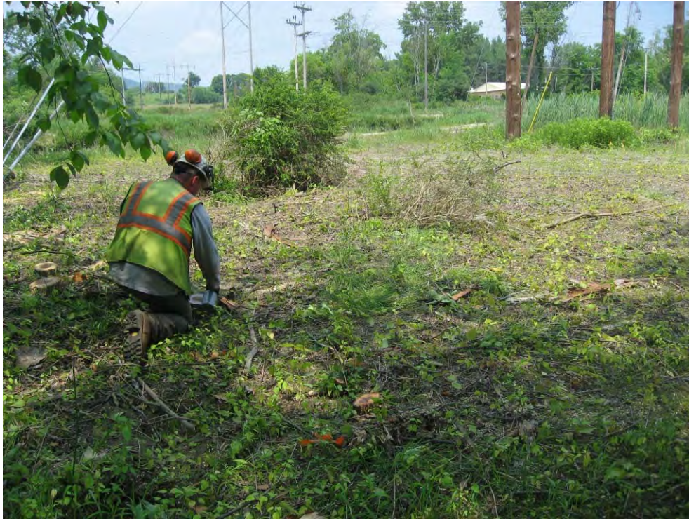
View of cut stump treatment with herbicide mix along K37 line.
