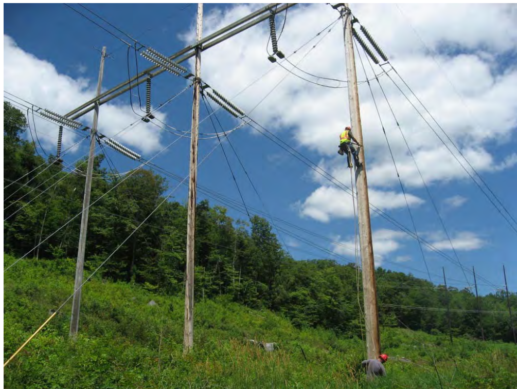
View of O&M crew climbing Structure 211 of the 340 Line to cut and top the wooden pole. No soil disturbance was observed or expected to occur.
